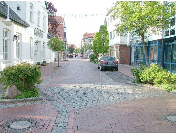
Sample Paving Detail creating Traffic Calming
